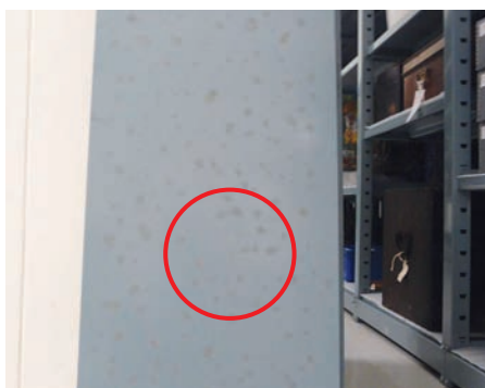
Figure 2. Rusted shelves. Photo courtesy of Alvin Tee
