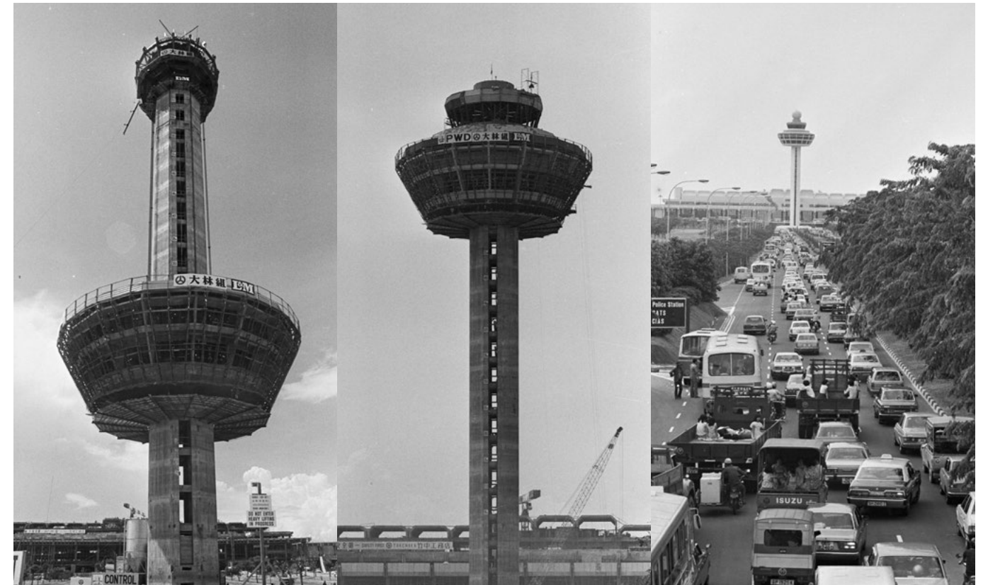
Sequence of construction of Changi Airport's iconic control tower, which was completed during Phase One of the airport's development. 1981. Photos: [L-R] Wong Kwai Chow, Tan Wee Him, Chew Yen Fook / The Straits Times
