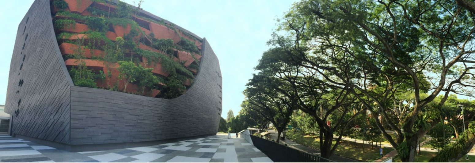
Façade and exterior of museum Photo courtesy of Lee Kong Chian Natural History Museum
