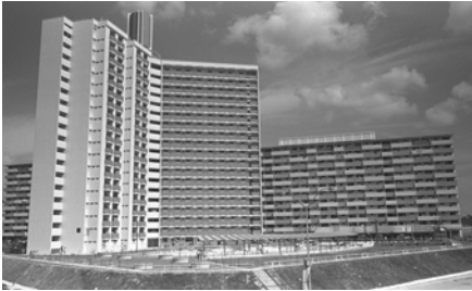
Y-shaped Block 53 with Blocks 54 and 55 in the background, 1967 Ministry of Information and the Arts Collection, courtesy of National Archives of Singapore
