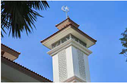
Double-tiered roof of the minaret which features ochre tiles, a hallmark of Malay architecture, 2022 Courtesy of National Heritage Board
