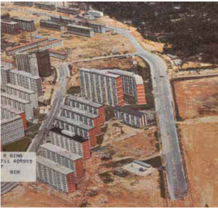
HDB blocks along Lorong 5 and Lorong 6 under construction, 1966 Courtesy of Housing & Development Board
