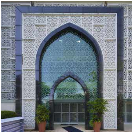
Entrance of the mosque combining several forms of Islamic architecture, including a rectangular frame, archways and a façade of geometric motifs with stylised floral patterns that recall traditional jali screens in Mughal architecture, 2022 Courtesy of National Heritage Board
