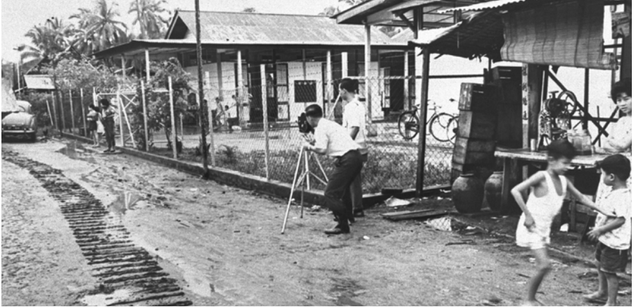
HDB official during earth-moving operations in a Toa Payoh kampong, 1963 Courtesy of National Archives of Singapore
