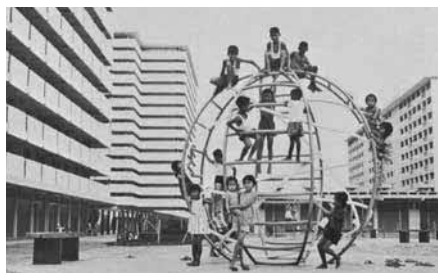
Early steel globe playground in Toa Payoh, 1969 Courtesy of Housing & Development Board
