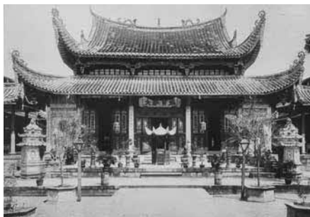
Double-tiered roofs of Mahavira Hall incorporate Fuzhou and Quanzhou architectural styles, 1950s Lee Kip Lin Collection, courtesy of National Archives of Singapore
