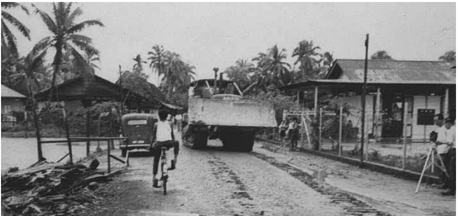
Kampong road in Toa Payoh made from macadam, which was an improvement on the laterite paths of the past, 1963 Courtesy of National Archives of Singapore
