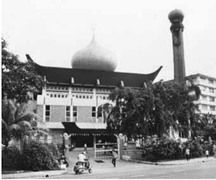
View of the original mosque from across Braddell Road, 1970s Majlis Ugama Islam Singapura Collection, courtesy of National Archives of Singapore
