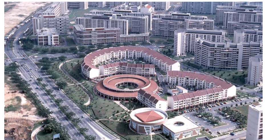
The low-rise Tampines Round Market and its high-rise surrounds, 1980s Courtesy of Housing & Development Board
