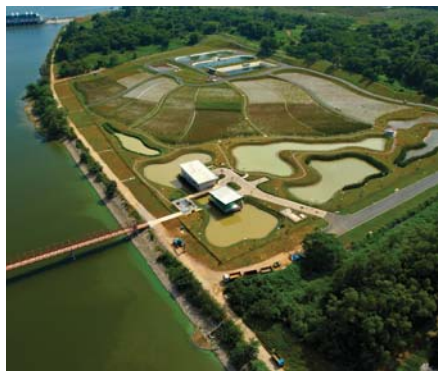
An aerial view of Lorong Halus Wetland, 2010 Courtesy of PUB, Singapore's National Water Agency
