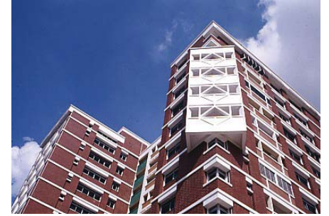
Projecting corner rooms of a HDB block in Tampines, 1992 Courtesy of Housing & Development Board
