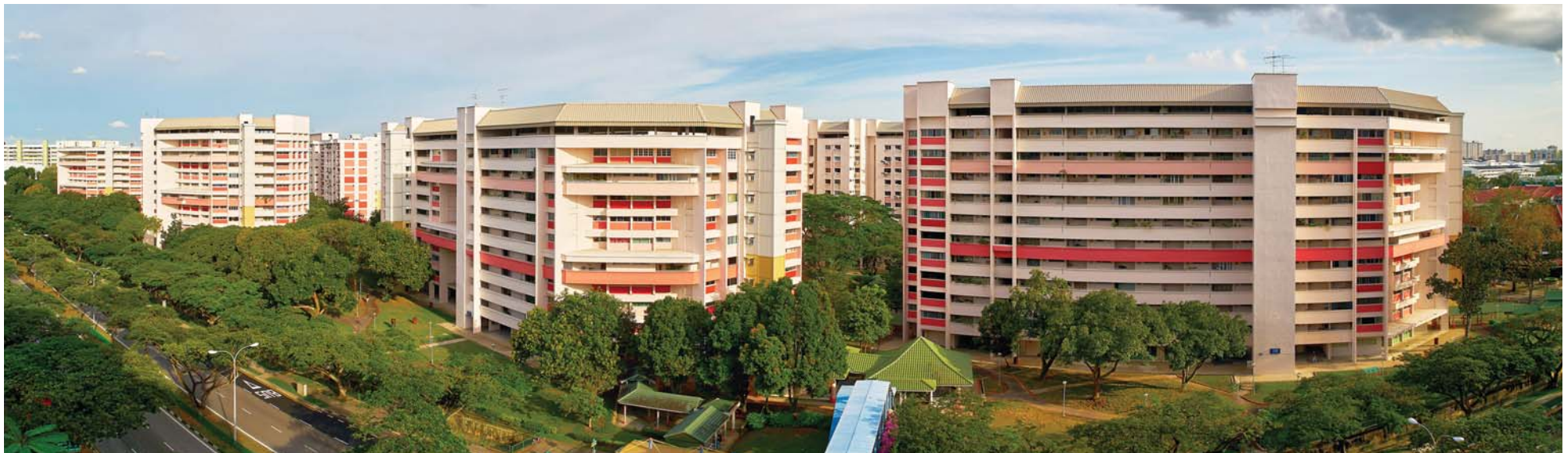
The earliest blocks of flats built in Tampines at Tampines Avenue 2, 2017 Courtesy of National Heritage Board
