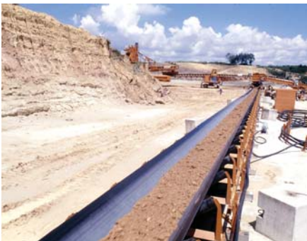
A conveyor belt transporting earth from Tampines to the eastern coast for reclamation, 1980 Courtesy of Housing & Development Board
