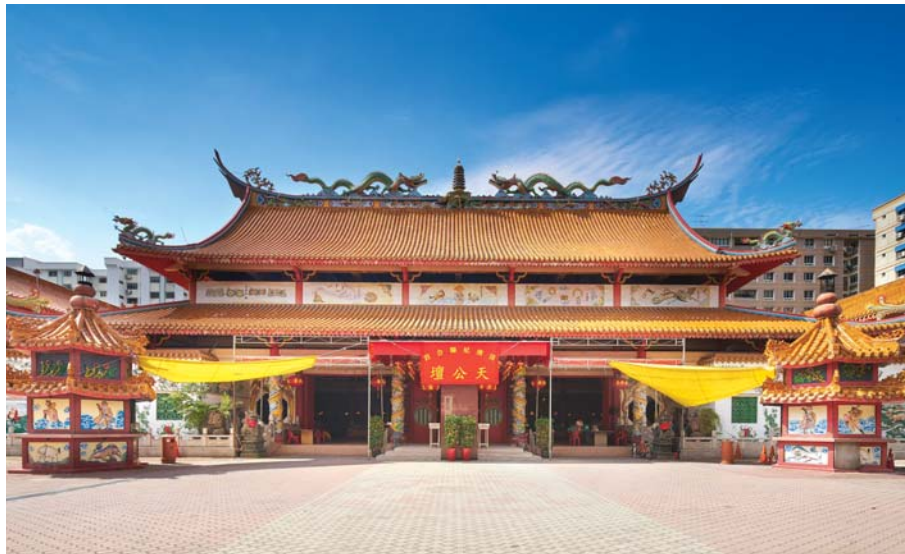
Tampines Chinese Temple, 2017 Courtesy of National Heritage Board
