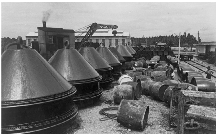
Floats and drums that support the boom nets at the Boom Defence Depot, 1941 © IWM (K 1302)
