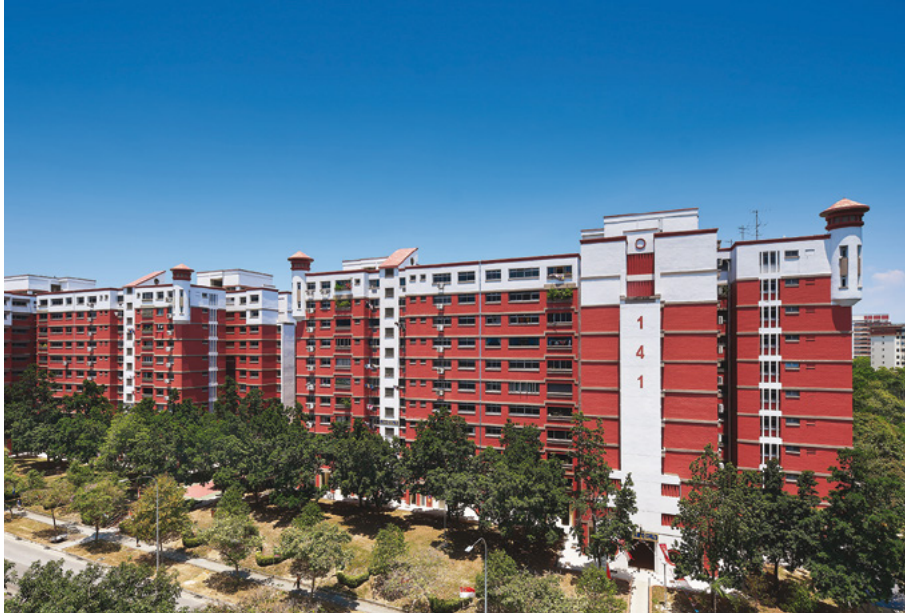
Flats with lighthouse-shaped turrets, 2019 Courtesy of National Heritage Board
