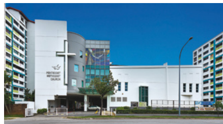
Pentecost Methodist Church, 2019 Courtesy of National Heritage Board
