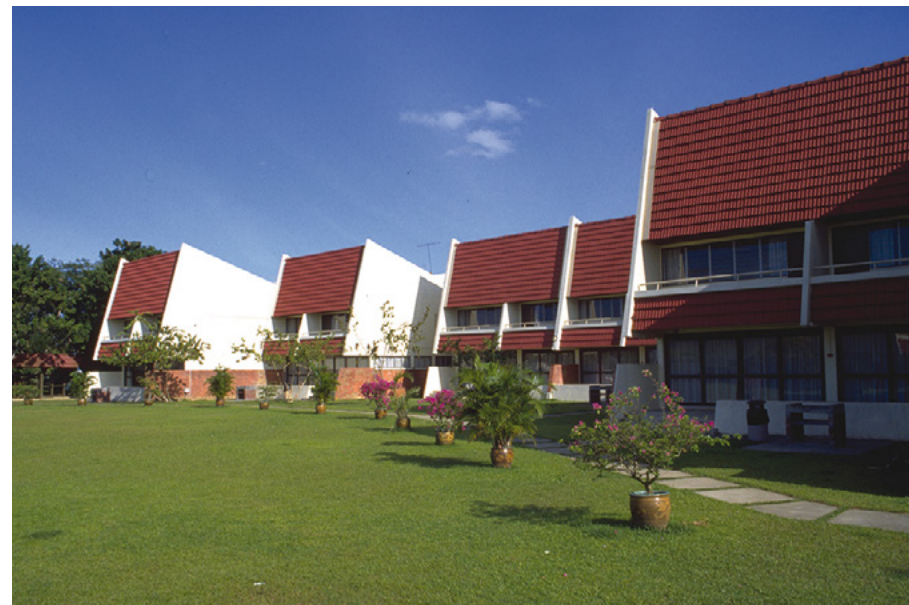
Holiday chalets built by the former Telecoms, 1987 Ministry of Information and the Arts Collection, courtesy of National Archives of Singapore
