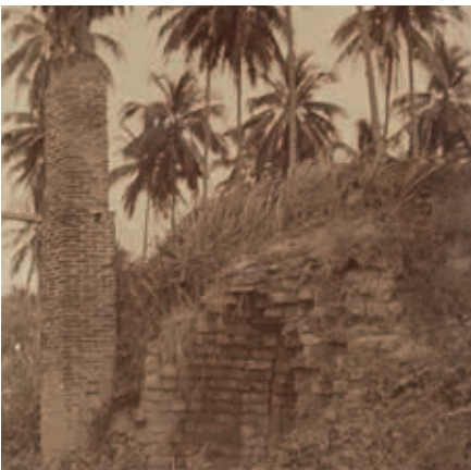
Photograph of an old brick kiln by Lim Lam San, c. 1930 Courtesy of National Museum of Singapore, National Heritage Board
