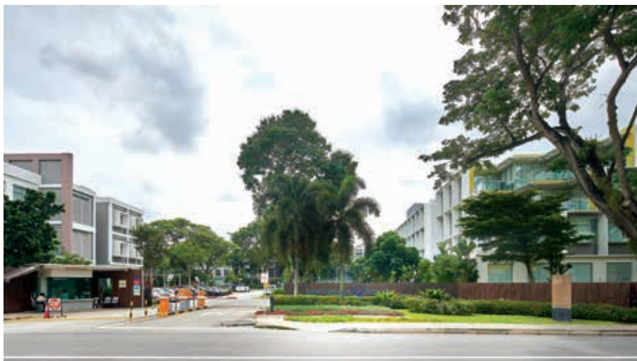
Site of Former KK Hospital (now Land Transport Authority Building), 2016
