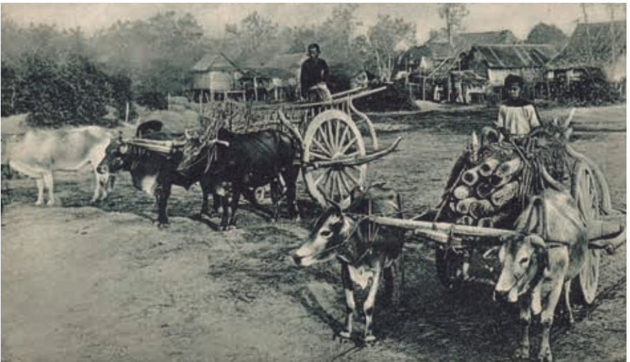
Postcard showing bullock carts being used to transport goods, late 19th century Courtesy of National Museum of Singapore, National Heritage Board
