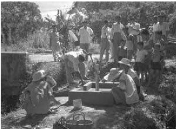
Workers installing a water standpipe in Jurong in 1959.
