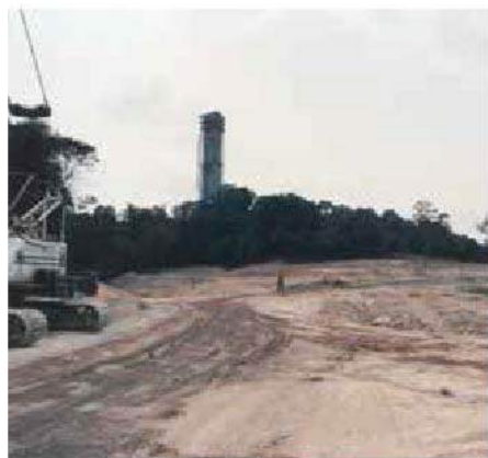
Starting construction works for the new SDC, 2005
