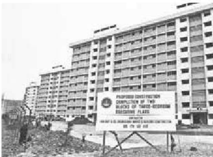
Three-room executive flats under construction in Jurong, 1973.
