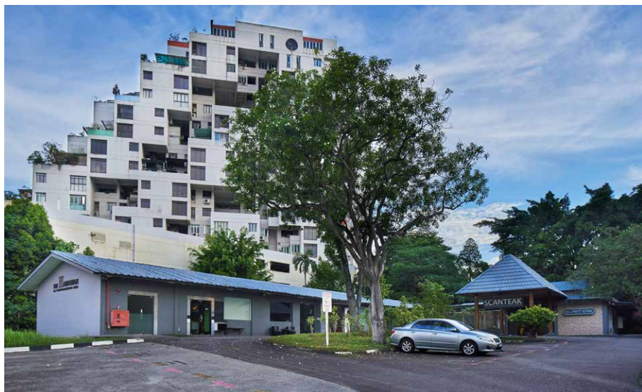
Former School Dental Clinic building, 2018
