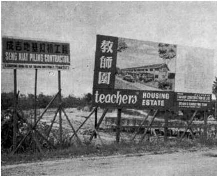
Signboard advertising the Teachers' Housing Estate at the construction site, 1968
