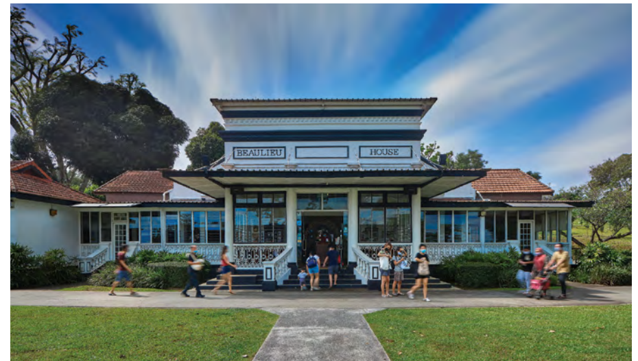
Beaulieu House, 2021 Courtesy of National Heritage Board
