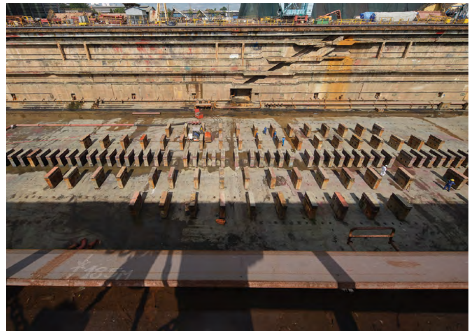
Rows of keel blocks (used to support a ship) at the bottom of King George VI Dry Dock, 2021 Courtesy of National Heritage Board
