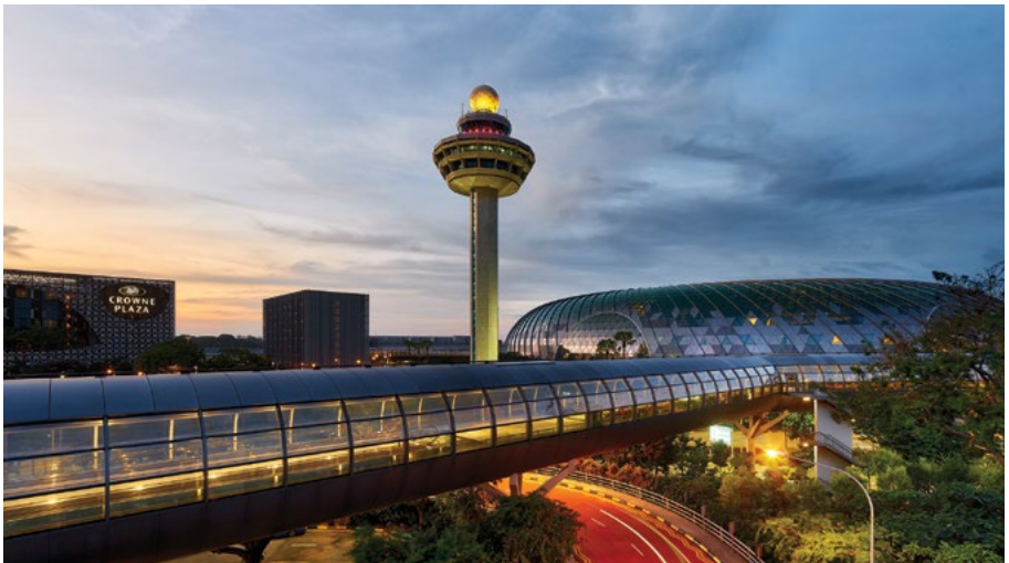
Changi Airport, 2024 Courtesy of National Heritage Board
