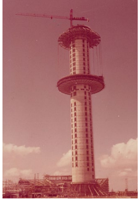
Changi Control Tower during its construction, 1979 Courtesy of Joshua Woo
