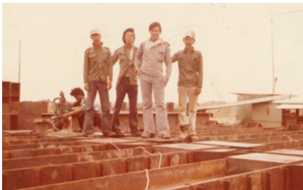
Woo Chee Yong and his colleagues at the construction site of Changi Control Tower, 1977 Courtesy of Joshua Woo
