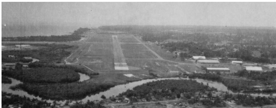
End of Changi Airport runway and Sungei Changi, 1965
