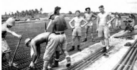
Japanese prisoners-of-war supervised by RAF personnel laying pierced steel planking runway of the Changi airfield, 1946
