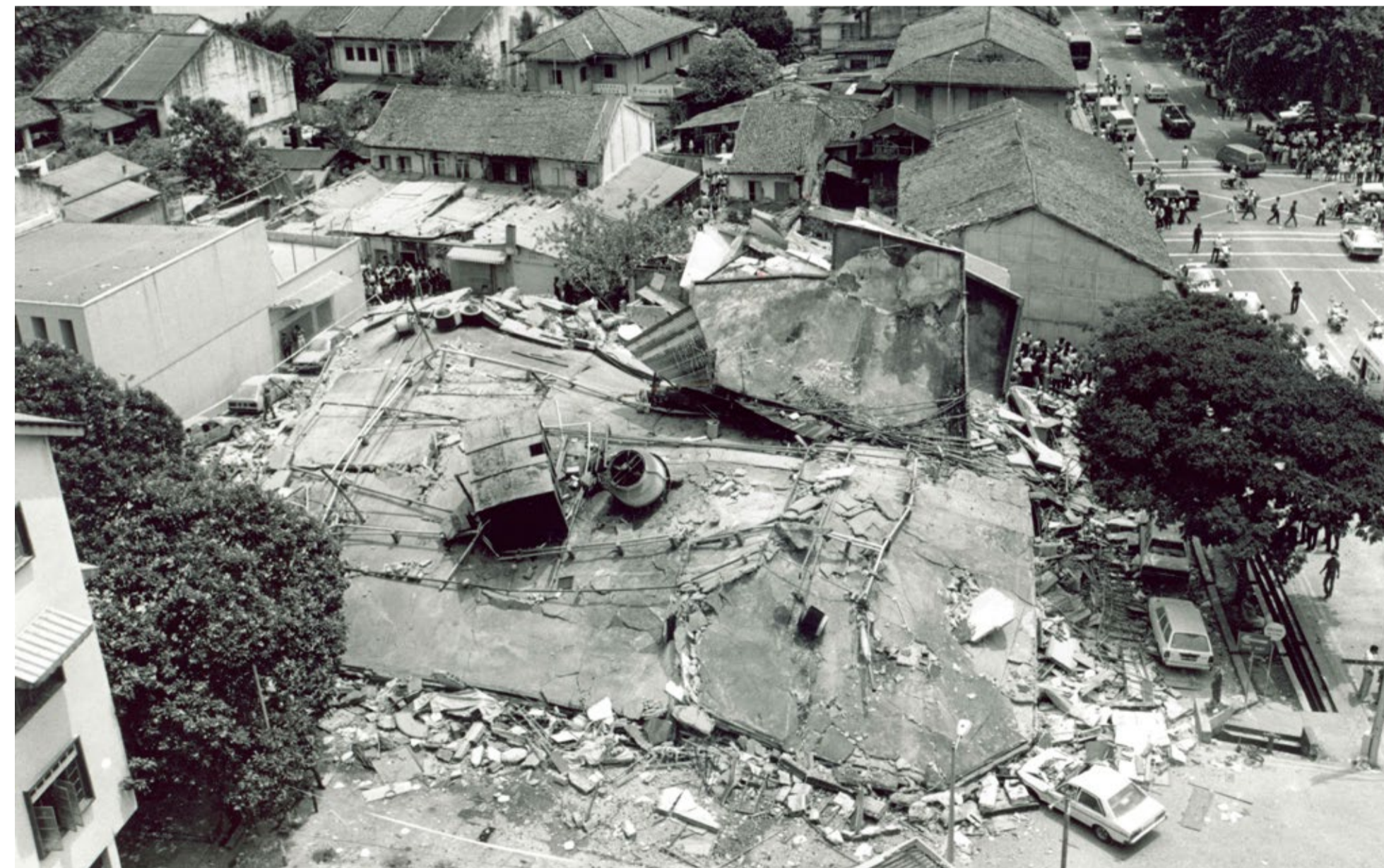
▲ An aerial overview of the Hotel New World collapse with the water tank and air conditioner compressor lying on top of the heap of debris (1986). Courtesy of Singapore Press Holdings
